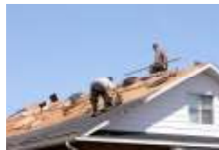
Typical work to be done on a Hearts for Homes project.
